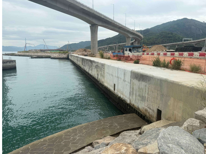
General View of Vertical Eco-shoreline
